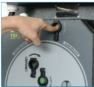
1 Open (OFF) the vacuum circuit-breaker
