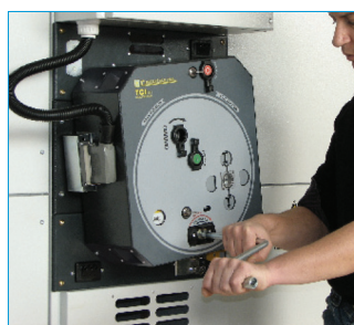
8 Lock the air rotary isolator in position "close"
