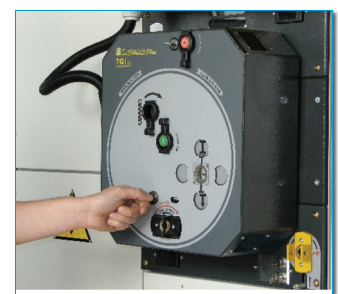
9 Lock the air isolator by the key (if available)
