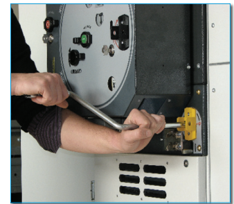
3 Open the earthing switch
