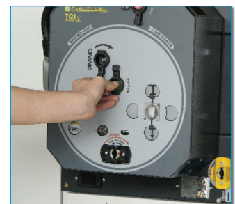
12 Close (ON) the vacuum circuit breaker
