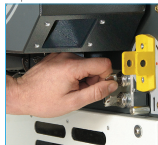
8 Unlock the earthing switch by the key (if available)
